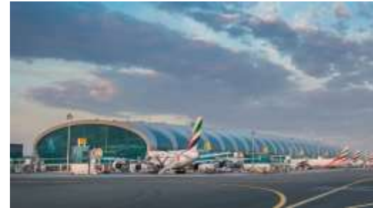
DUBAI AIRPORTS – TERMINAL 1 Special Airport Systems Installation
