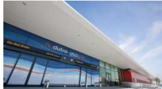
DUBAI AIRPORTS – TERMINAL 2 Special Airport Systems Installation
